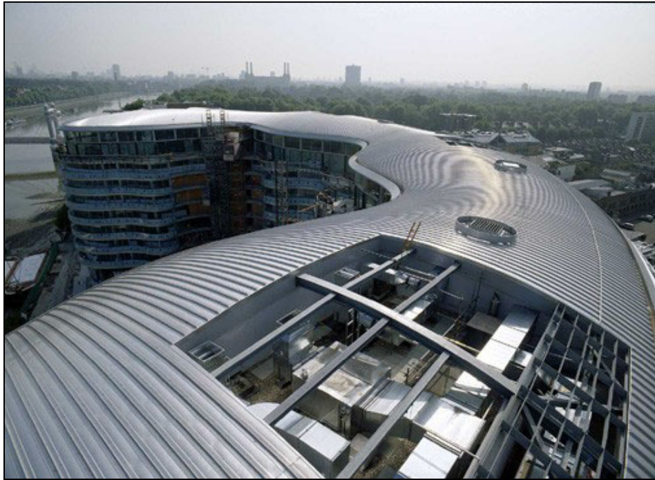
Figure 5.12 Kalzip ® roofing used at Albion Riverside, London (Courtesy of Kalzip ® )
