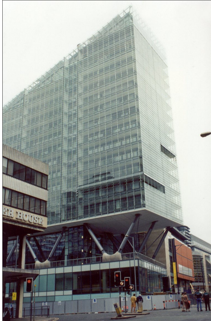
Figure 1.3 16-storey composite steel framed building in Manchester
