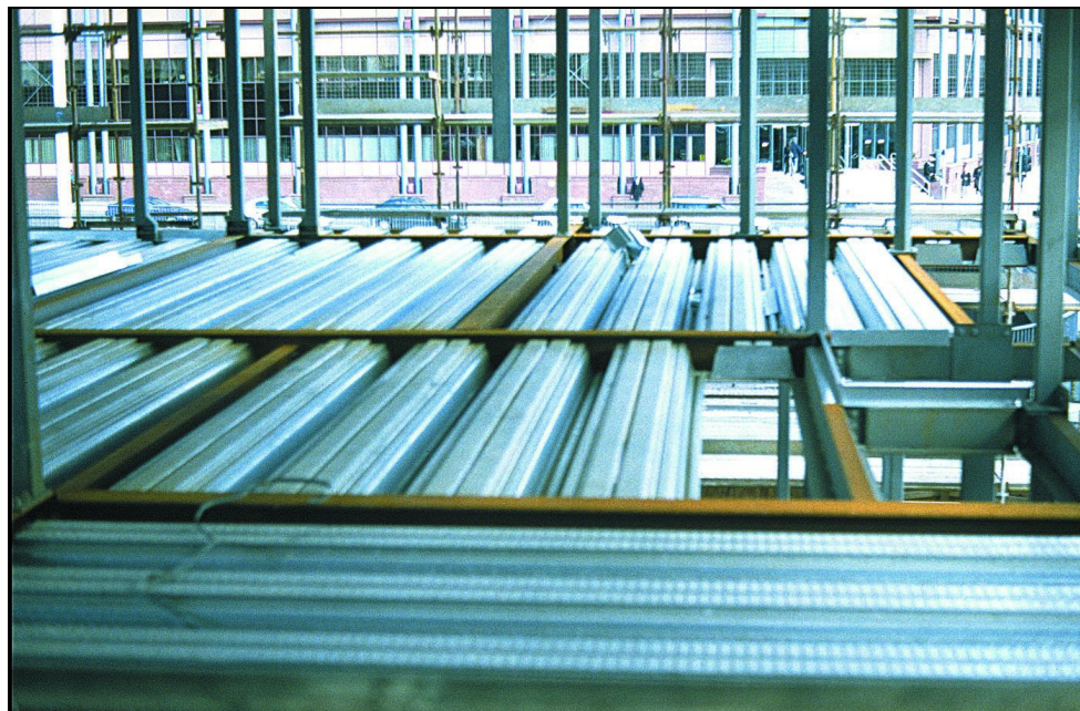
Figure 4.5 Slimdek and SHS columns used in a residential building
