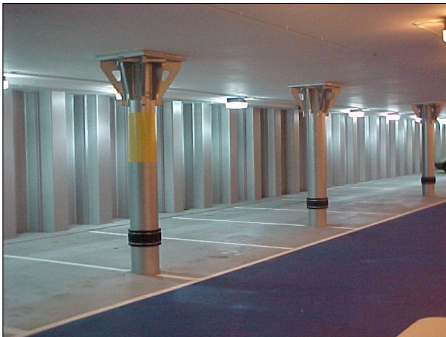
Figure 7.2 Millennium Car Park, Bristol showing sheet piling and the column head detail supporting the floor slab
