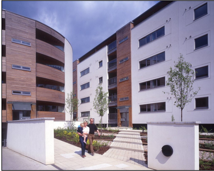
Figure 5.2 Insulated render used with timber cladding (Courtesy of Feilden Clegg Bradley)
