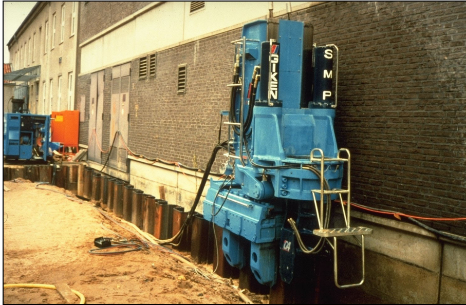
Figure 7.1 Silent piling machine
