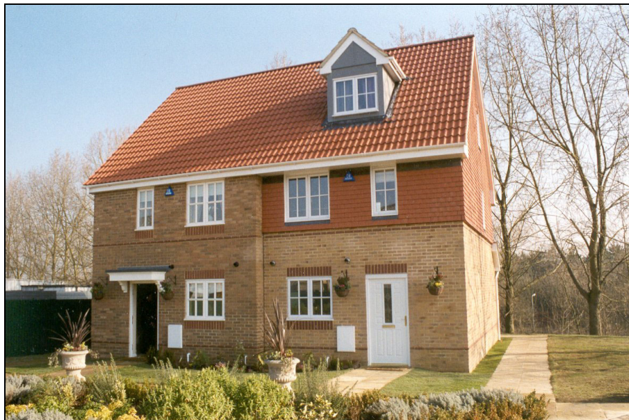
Figure 5.6 Brick-tiles used in a housing project
