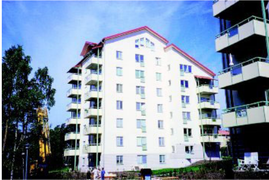
Figure 6.1 Stacked modular balconies (project in Sweden)
