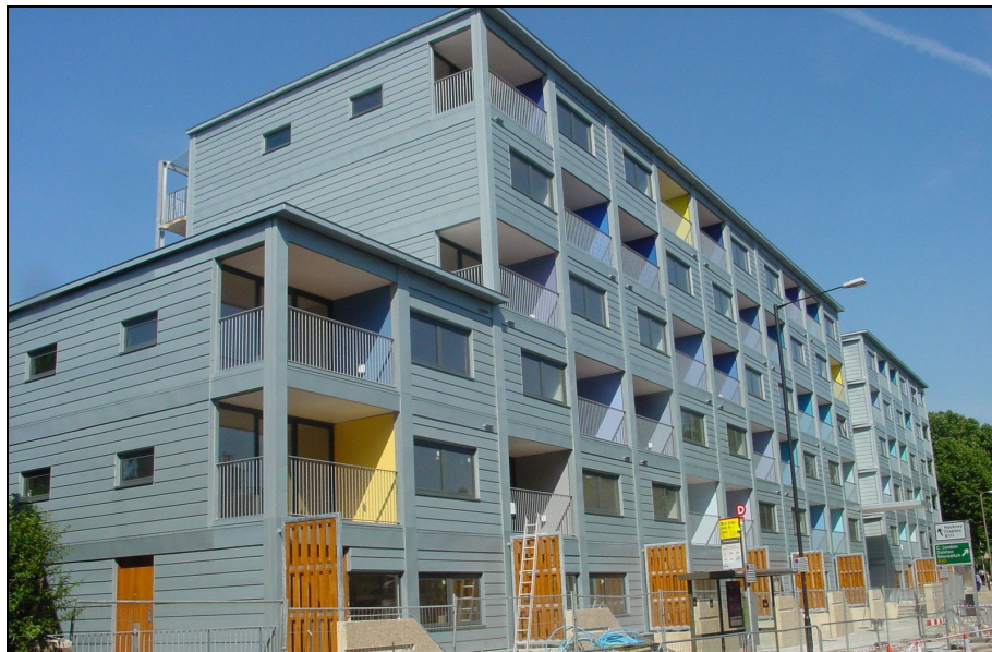
Figure 5.11 Zinc sheets used at Raines Court, London
