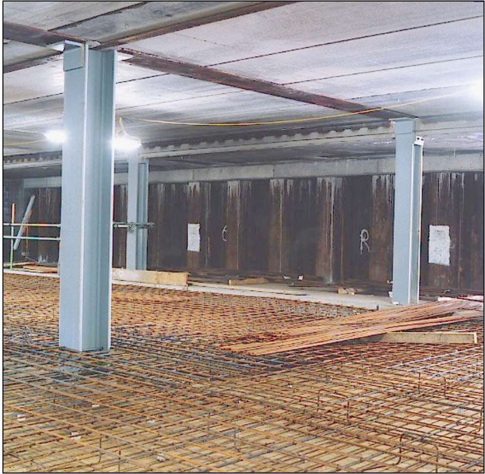
Figure 7.3 Use of Slimflor beams in basement construction
