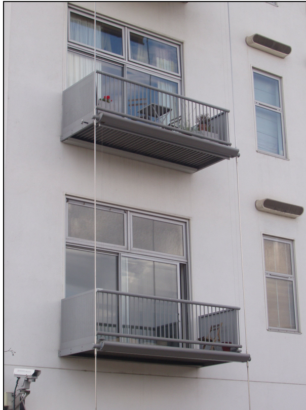
Figure 6.7 Suspended balconies (Piper Building, Fulham)
