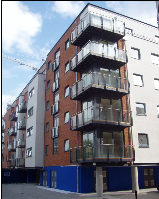
Figure 6.5 Corner cantilevered balconies at Admiral's Quay, Southampton (Courtesy of Broadway Malyan)
