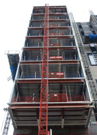
Feature elements: One of the structure's two cantilevers
