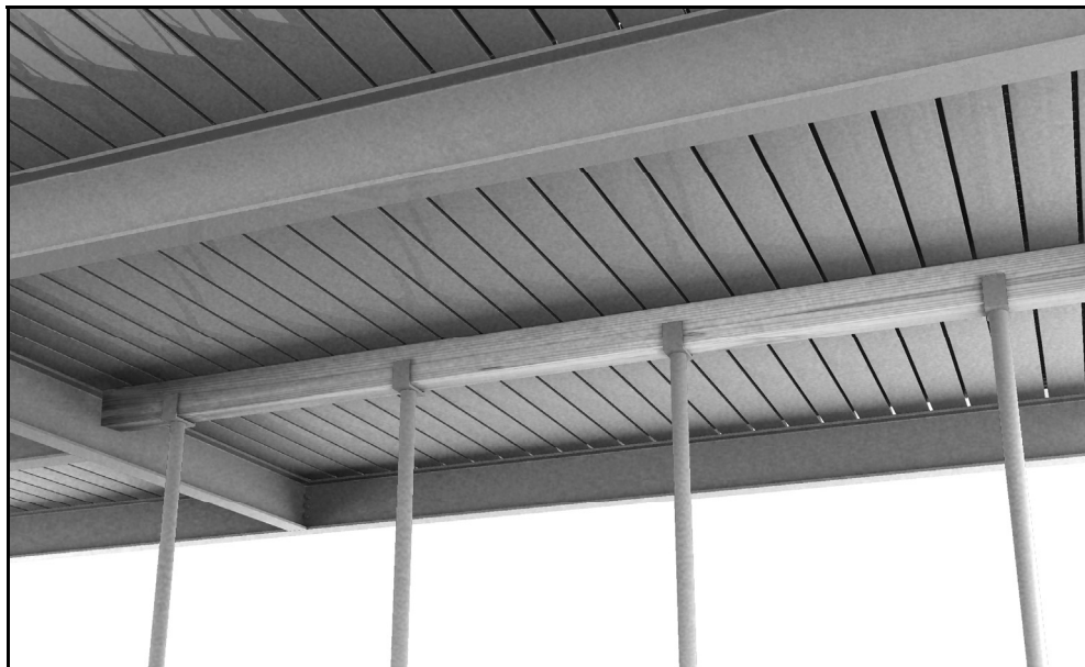
Figure 4.17 Temporary support using an 'Acrow' props
