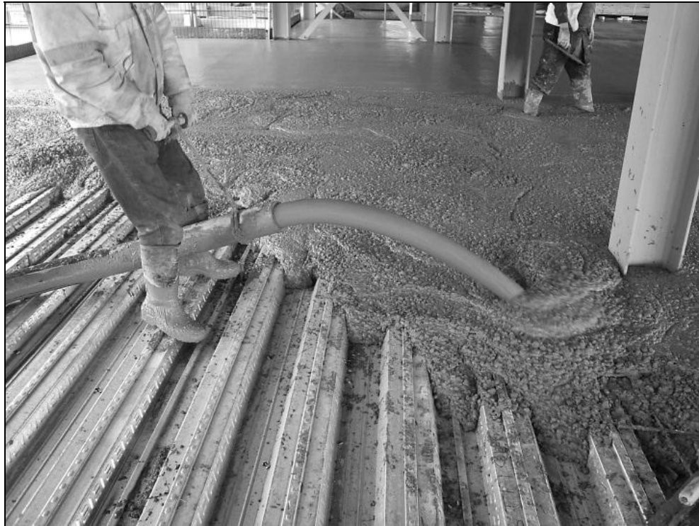
Figure 6.4 Pumping of fibre-reinforced concrete
