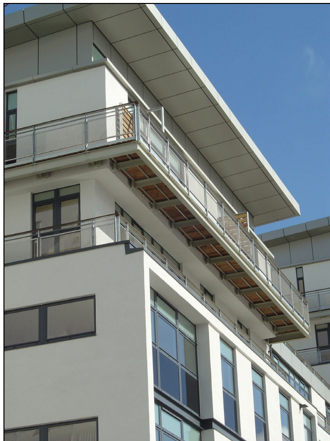
Figure 3.4 Details of insulated render cladding at parapet and balcony - Cala House, Glasgow
