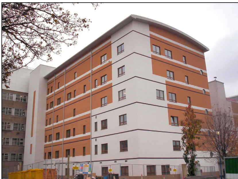
Figure 3.5 Insulated render used in multi-storey building at Sunderland Royal Hospital showing detailing at floor lines
