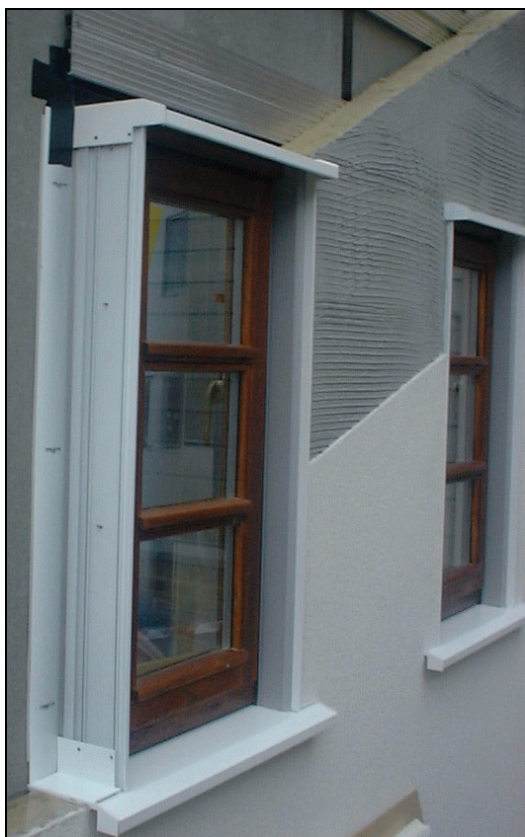
Figure 3.2 Window pod detail and wall build-up
