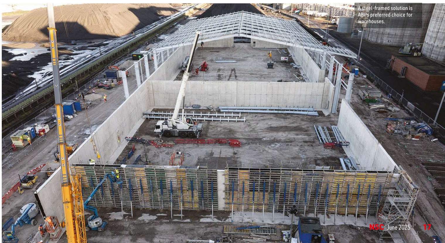
Steel canopies cantilever over the warehouse's entrances.
