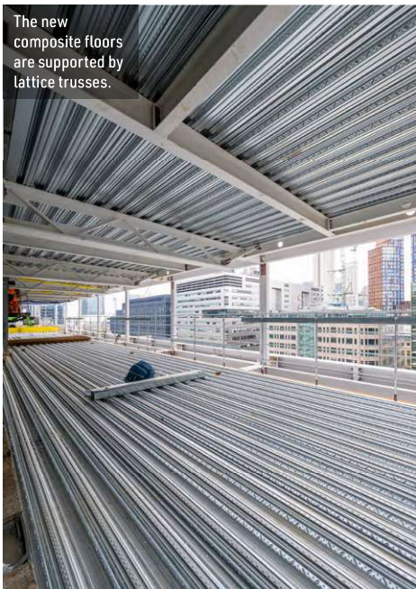
Infilled areas have used beams with cellular openings to accommodate the building's services.
