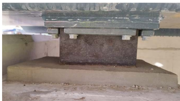
Figure 6 Proprietary designed elastomeric Type 1.1 free bearing beneath steel bridge deck (note bolted ‘keep’ plates to top plate to reduce risk of bearing moving out over time)
