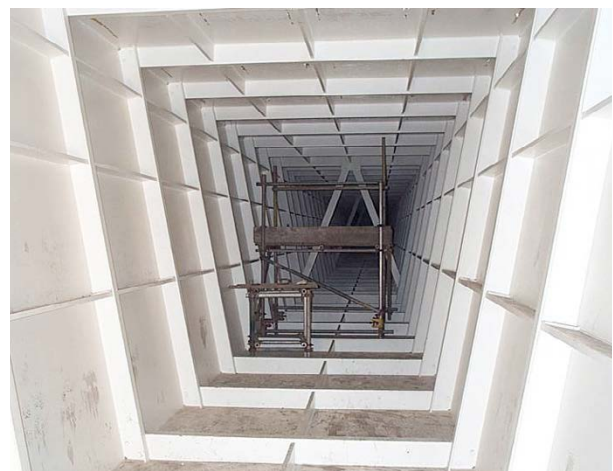
Figure 1 Internal view of a steel box girder showing use of longitudinal stiffeners
