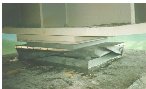
Figure 3 Guided bearing (with skirt)
