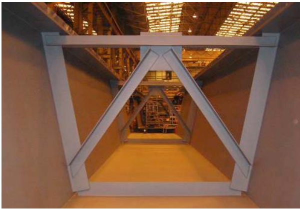
Figure 2 Internal view of a steel box girder where longitudinal stiffeners were avoided by the use of thicker plates
