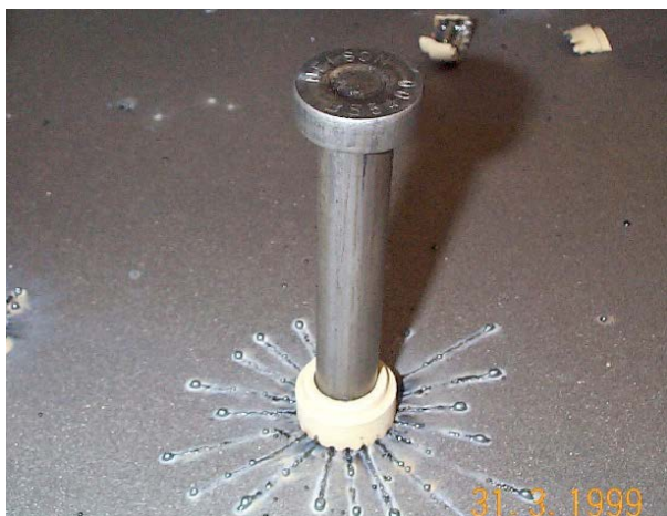
Figure 3 Typical shear stud after welding
