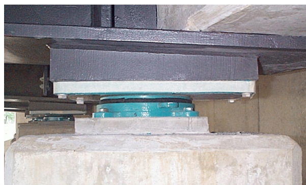
Figure 2 Attachment by bolts in tapped holes (bearing plate is welded to flange)
